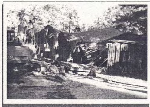
Tearing down the old Dining Hall.
